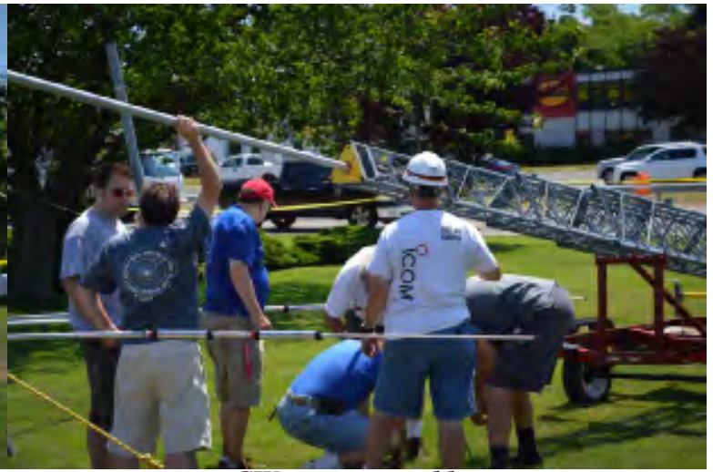
CW tower assembly
