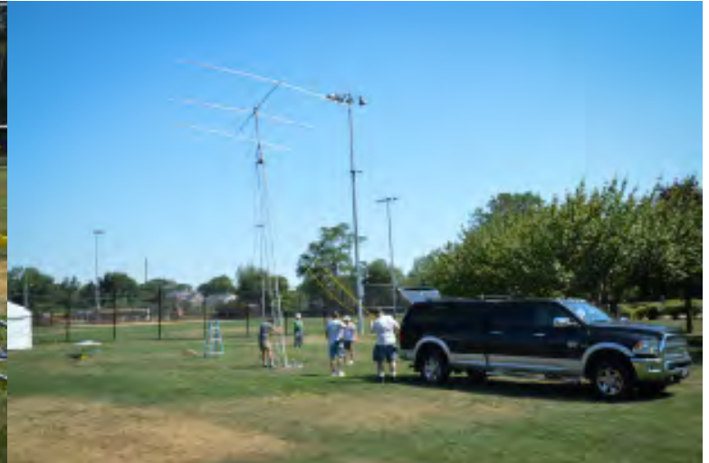
The SSB Tribander is raised
